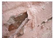
These photographs show where saponification has occurred and the binder in the paints has been broken down resulting in unsightly paint failure.
